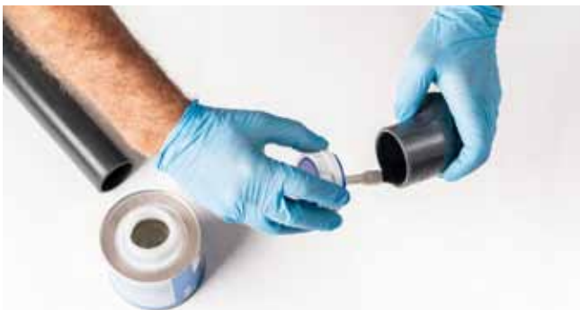
Apply a normal layer of adhesive and cover the fitting axially
