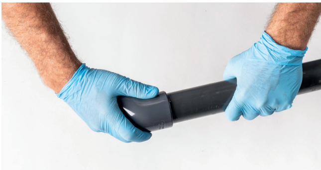
Fully insert the pipe into the fitting immediately and apply pressure to the joined parts. Then use paper or cloth to remove any excess solvent cement from the outer surfaces
