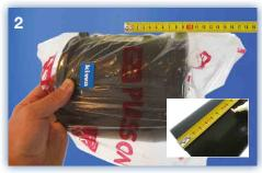
2. Measure the insertion depth of the fitting. Add 20mm and mark this length on the pipe end, using a white marker.
