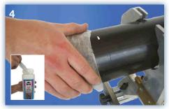
4. Clean pipe ends with authorized cleaner to remove any dirt, and allow to dry. Only use a wipe once. Do not touch the prepared surfaces.
