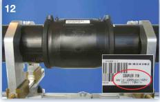
12. Leave the joint in the clamps to cool. Do not pressurize the system before cooling time X3 has passed
