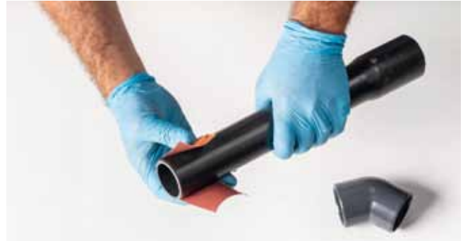
Sand slightly to make the surfaces to be glued dull
