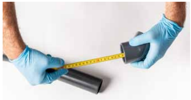
Leave the surfaces to dry for a few minutes before applying the solvent cement. Measure the pipe insertion length and mark this length at the end of the pipe
